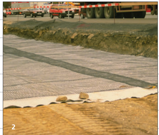
Photo 1 + 2: Base reinforcement with Fornit® geogrids.
