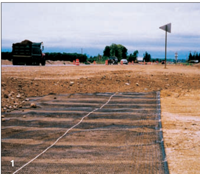
Photo 1 + 2: Base reinforcement with Fornit® geogrids.
