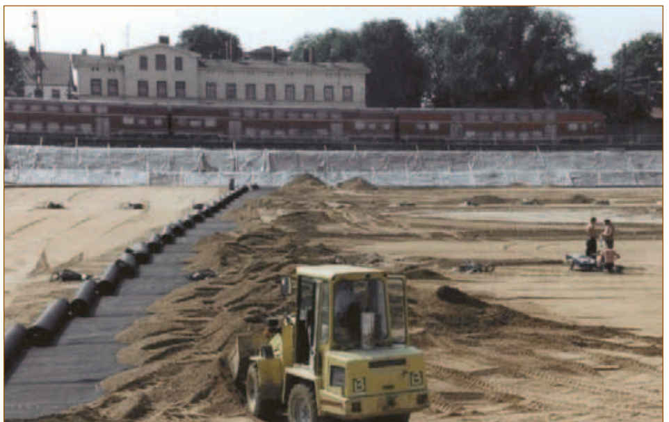
Ensuring safety of a railway junction in the former mining area of Gröbers
