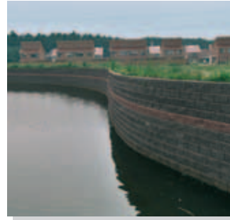
Segmental Retaining walls
