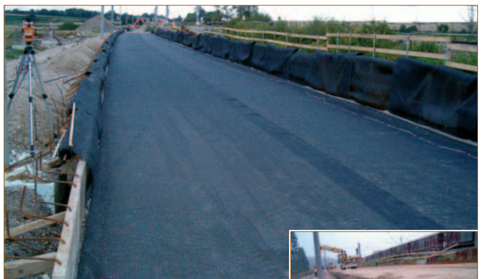
Railway embankment on piles, Augsburg-Olching Project
